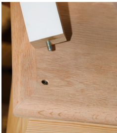
Treads are drilled for balusters, and inserts are installed.
