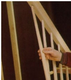
Rake rails on stair are drilled for easy baluster insertion, up into rail and down into tread.
