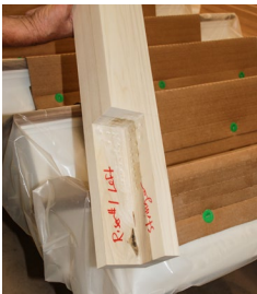
Post is notched for exact location and height.
