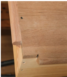
Stair is notched for post.
