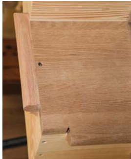
Stair is notched for post.
