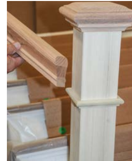
One end of rail is precut for quick field installation with post to post rail systems. Opposite end is cut to fit in field.
